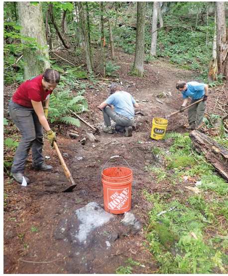
From left: Tyler installing bridge decking; Seasonal Trail Crew staff bench cutting new trail and building water bars; Ernie the Gurney is a two person rock carrier, built by Tyler.
