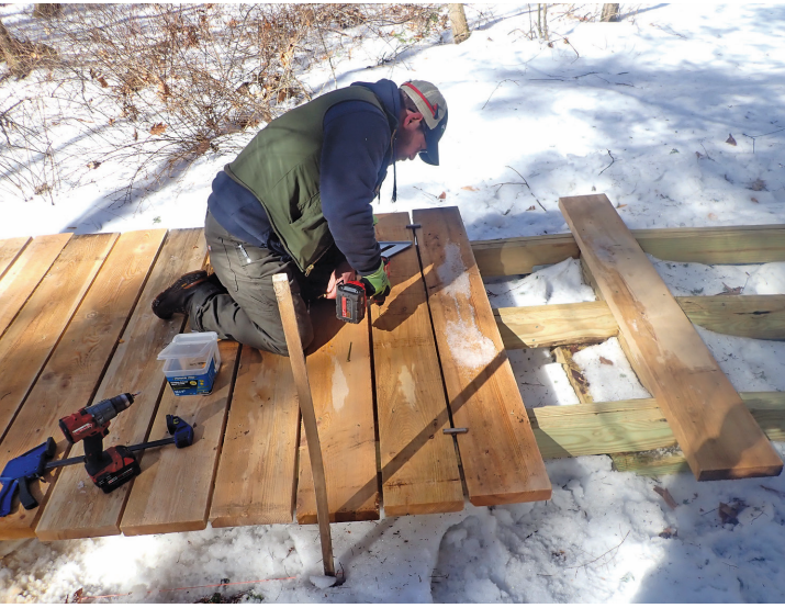
From left: Tyler installing bridge decking; Seasonal Trail Crew staff bench cutting new trail and building water bars; Ernie the Gurney is a two person rock carrier, built by Tyler.
